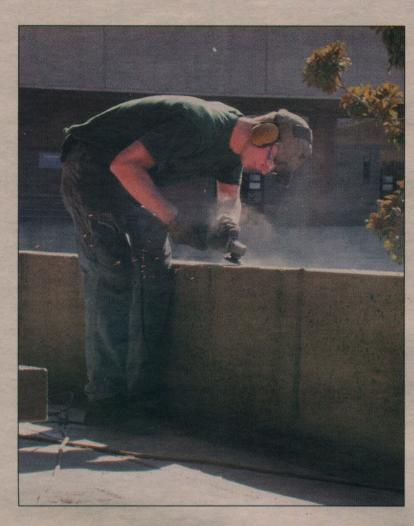
Ben Jablonski, an LB student working for TK Fabrications, grinds down the brackets in preperation for a new iron railing to replace the old wooden rails.
