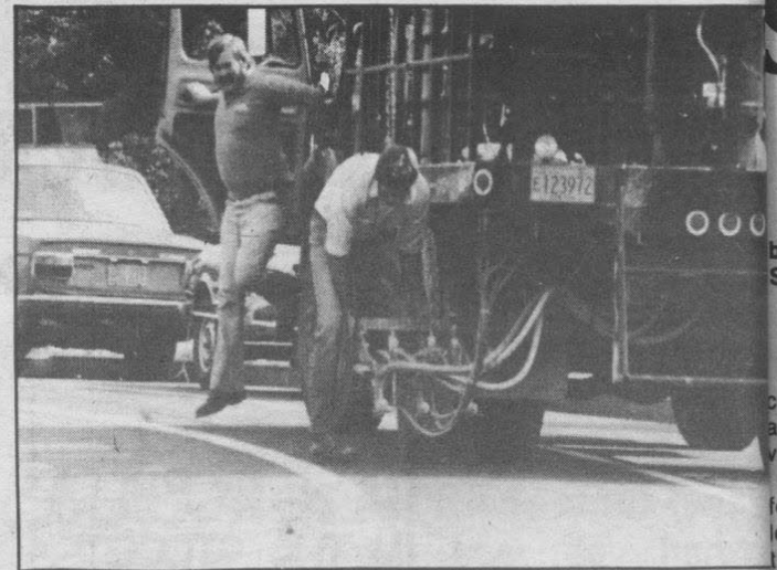
Workmen paint bike lanes on Corvallis street.
