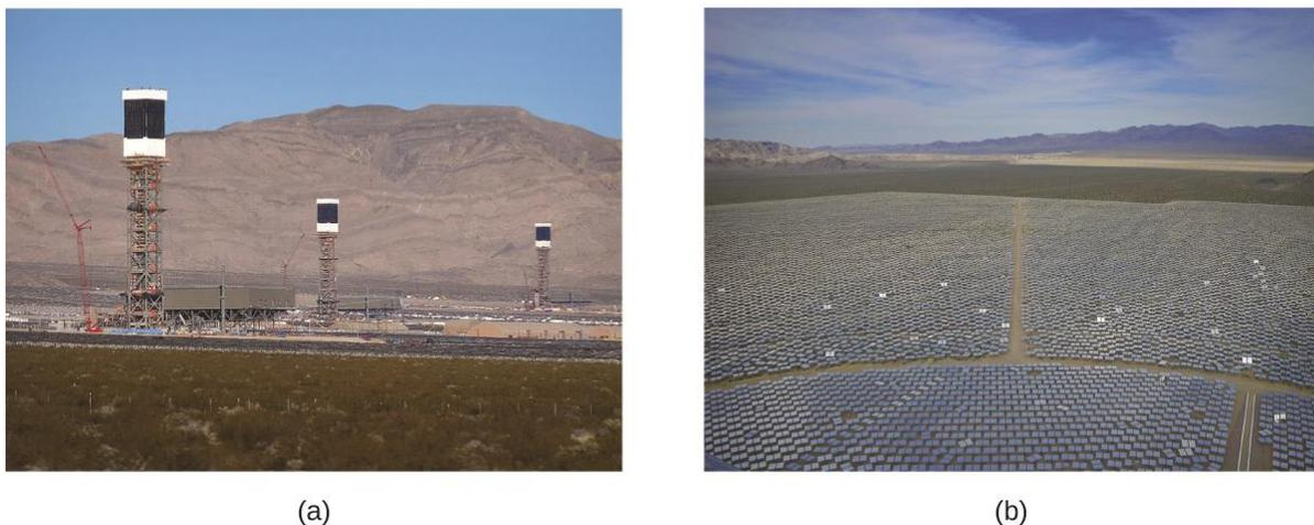
**Figure 8.11** (a) The Ivanpah solar thermal plant uses 170,000 mirrors to concentrate sunlight on water-filled towers. (b) It covers 4000 acres of public land near the Mojave Desert and the California-Nevada border. (credit a: modification of work by Craig Dietrich; credit b: modification of work by “USFWS Pacific Southwest Region”/Flickr)
