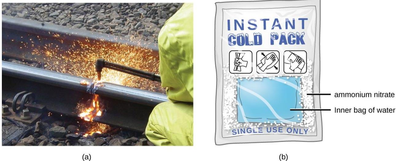
**Figure 8.8** (a) An oxyacetylene torch produces heat by the combustion of acetylene in oxygen. The energy released by this exothermic reaction heats and then melts the metal being cut. The sparks are tiny bits of the molten metal flying away. (b) A cold pack uses an endothermic process to create the sensation of cold. (credit a: modification of work by “Skatebiker”/Wikimedia commons)
