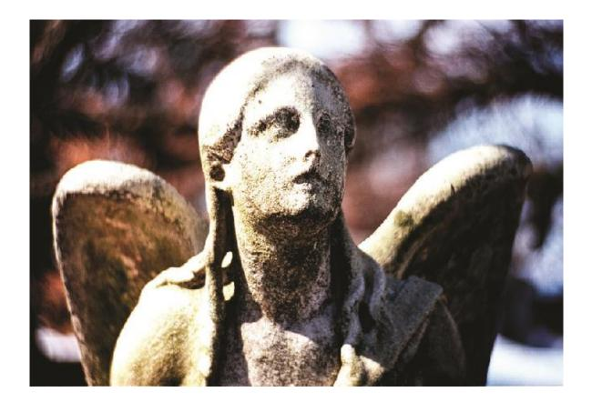
**Figure 12.7** Statues made from carbonate compounds such as limestone and marble typically weather slowly over time due to the actions of water, and thermal expansion and contraction. However, pollutants like sulfur dioxide can accelerate weathering. As the concentration of air pollutants increases, deterioration of limestone occurs more rapidly. (credit: James P Fisher III)
