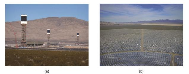
**Figure 8.11** (a) The Ivanpah solar thermal plant uses 170,000 mirrors to concentrate sunlight on water-filled towers. (b) It covers 4000 acres of public land near the Mojave Desert and the California-Nevada border. (credit a: modification of work by Craig Dietrich; credit b: modification of work by "USFWS Pacific Southwest Region"/Flickr)
