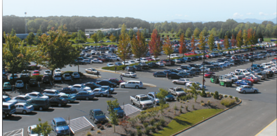
Aerial shot of LBCC's south lot.
