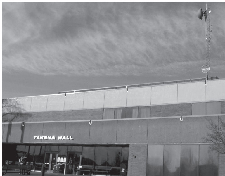
Takena Hall, home to one radio tower.
