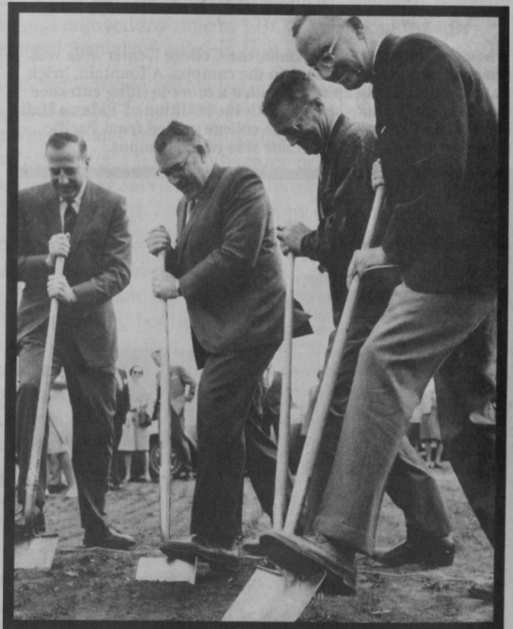
College administrators and college supporters take part in the ground breaking ceremony for the soon-to-be-constructed LBCC campus. Left to right are Russ Tripp, Dr. Eldon Shafer, Glen Huston and Dr. O. Robert Adams.
