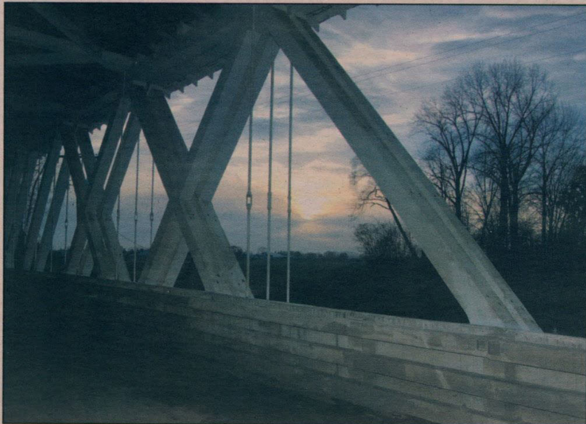
Above: The Truss-Howe design, of the Hoffman Bridge north of Crabtree on Hungry Hill Drive, is evident in this 90-foot span constructed in 1936.
