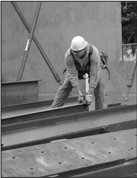
Construction workers put up interior steelwork
